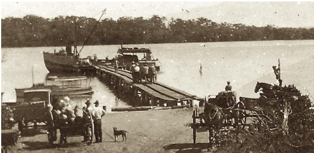
Figure 22. Russell Island jetty ca 1920s. Photo credit: Peter Ludlow.
