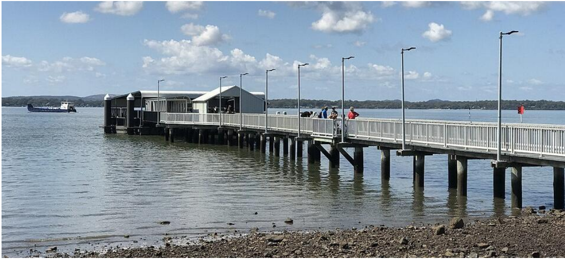
Figure 26. Victoria Point ferry terminal jetty. Photo credit: Redland City Council.
