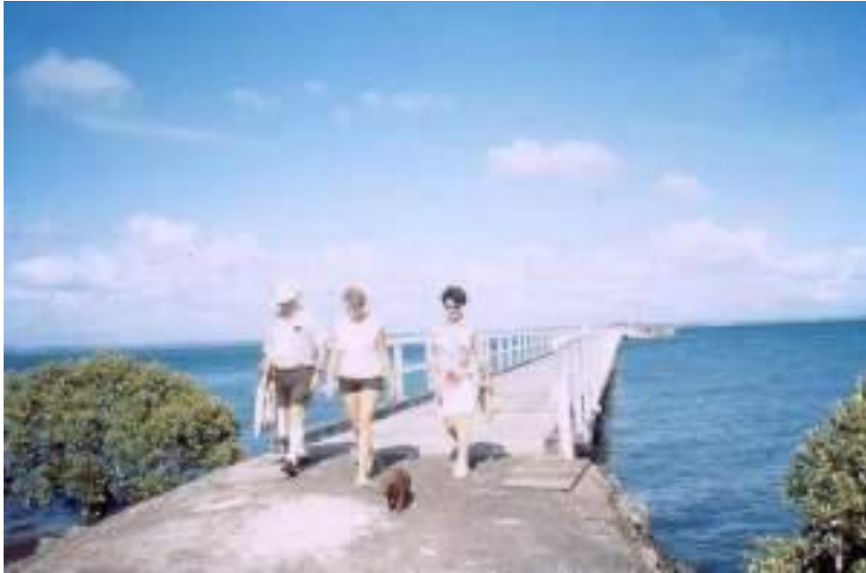
Figure 12. The Queensland Government Peel Island western jetty in 1990. Photo credit: Peter Ludlow.
